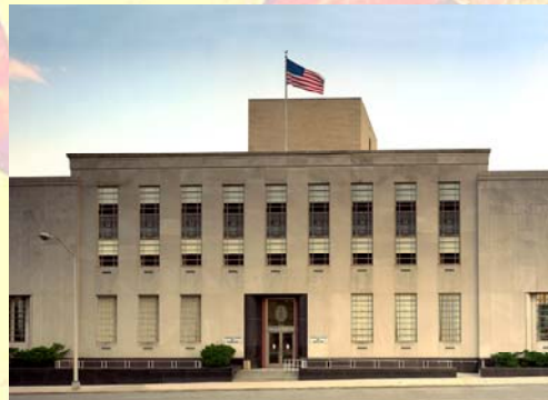
District Court in Baltimore, MD (Fayette Location)
